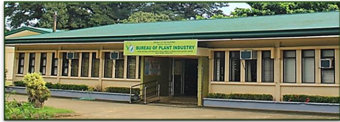
Figure 45. Davao National Crop Research, Development and Production Support Center (DNCRDPSC).
